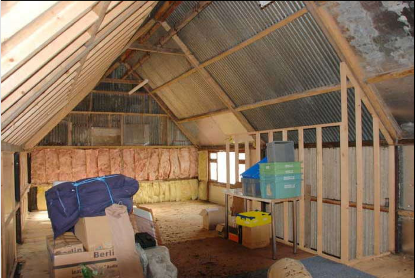
Loft Room in the G.P. Building
