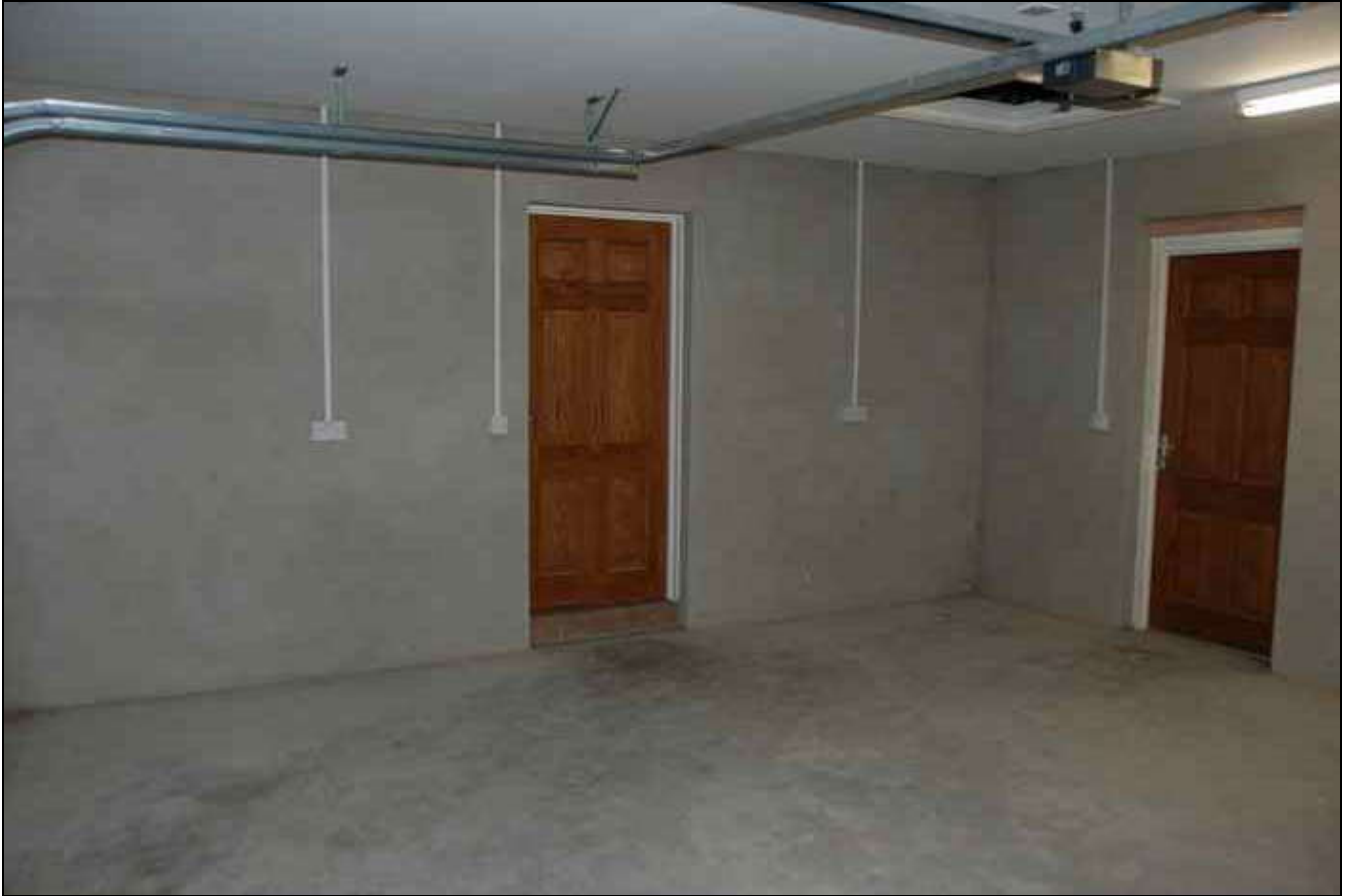
Inside the Garage
