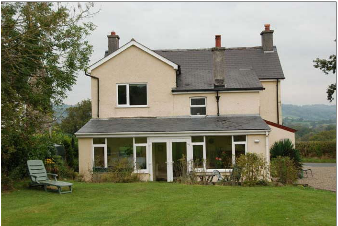
Rear View of the House
