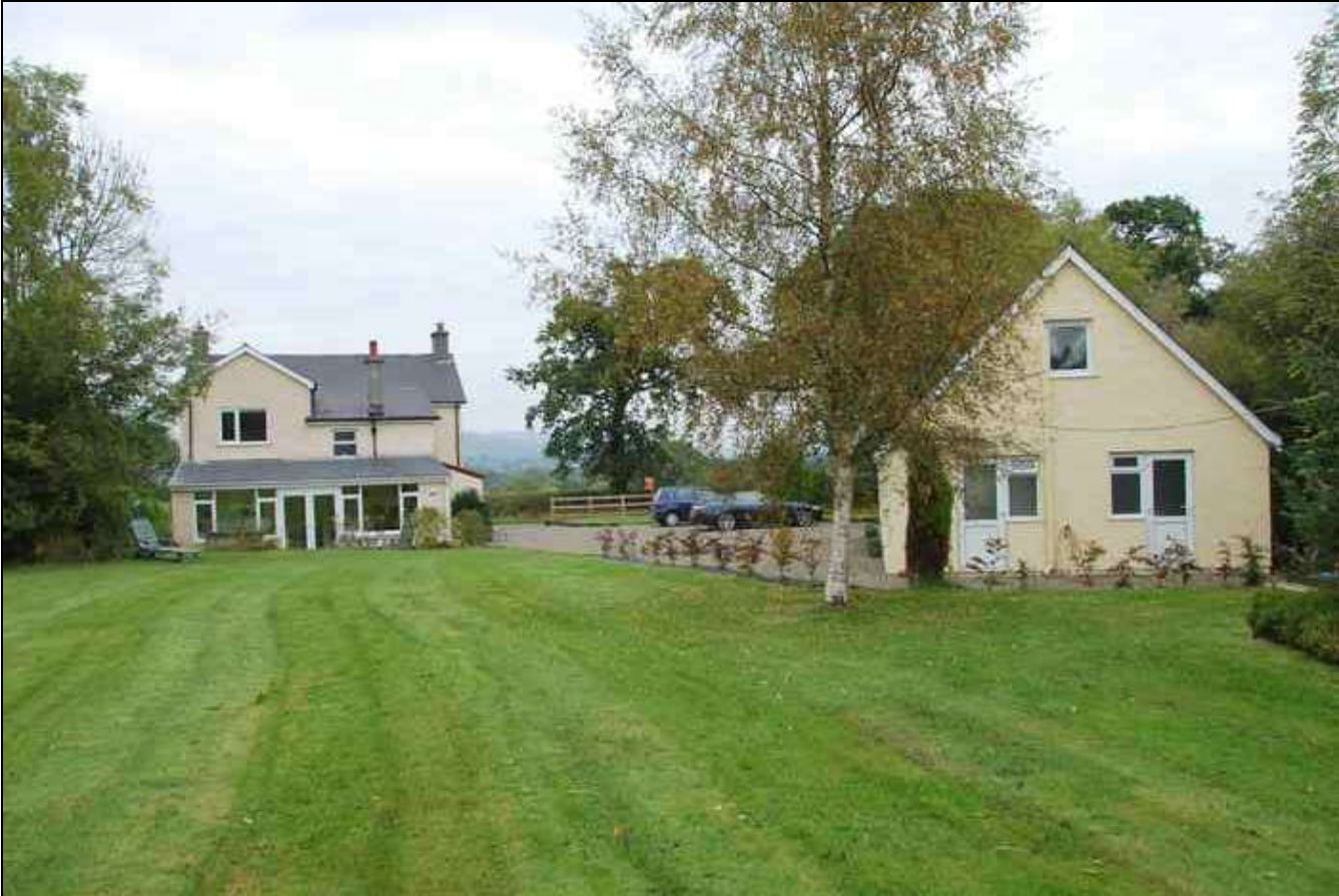
A rear view of the house and garage outbuilding (with scope for conversion subject to planning consent)
