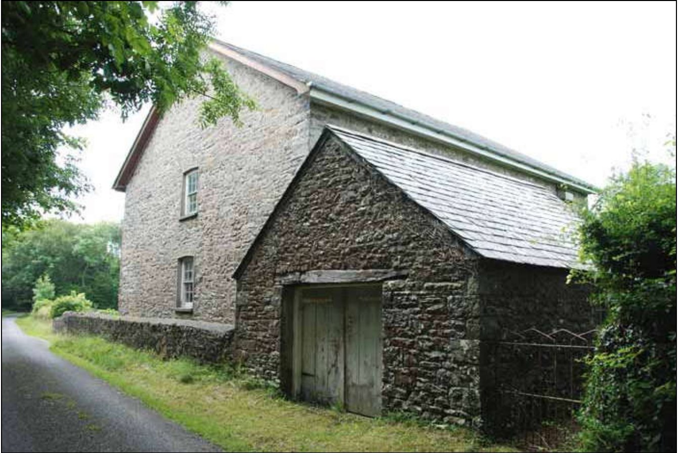
The stone outbuilding behind the chapel
